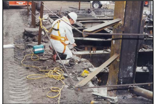
A metallurgical engineer evaluates damage effects at an accident site
