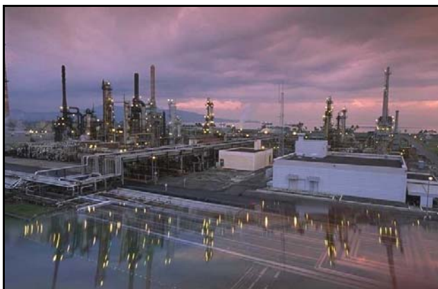
Pressure vessels, piping and pumps are assessed for corrosion and high temperature damage to maintain safe plant operations
