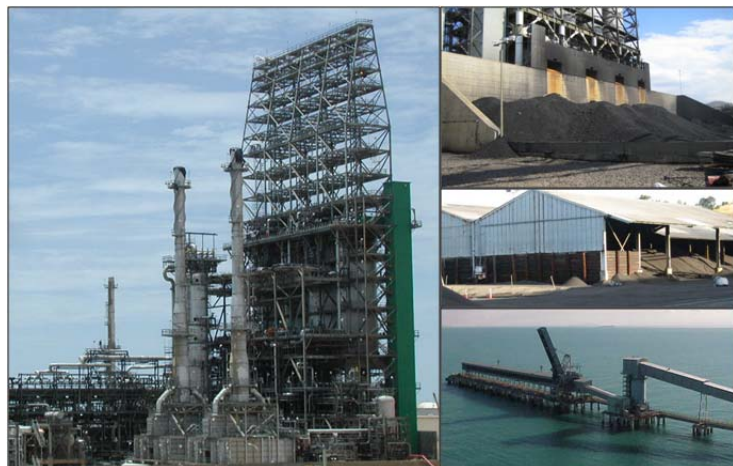
Typical Delayed Coking Unit and Coke Distribution Facilities
